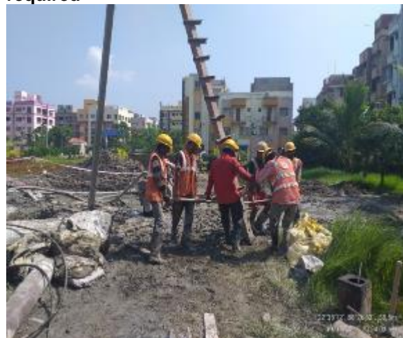
Partial use of safety gears seen in piling activity
